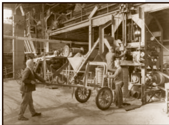
Early McCracken Model E pipe machine producing bell down concrete pipe.
