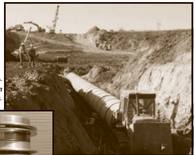
Job site view of a large-bore concrete pipeline in an open trench installation.
