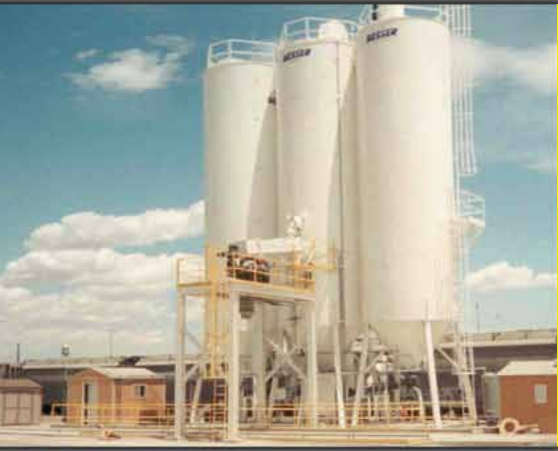
Easy tank cement load-out terminal
