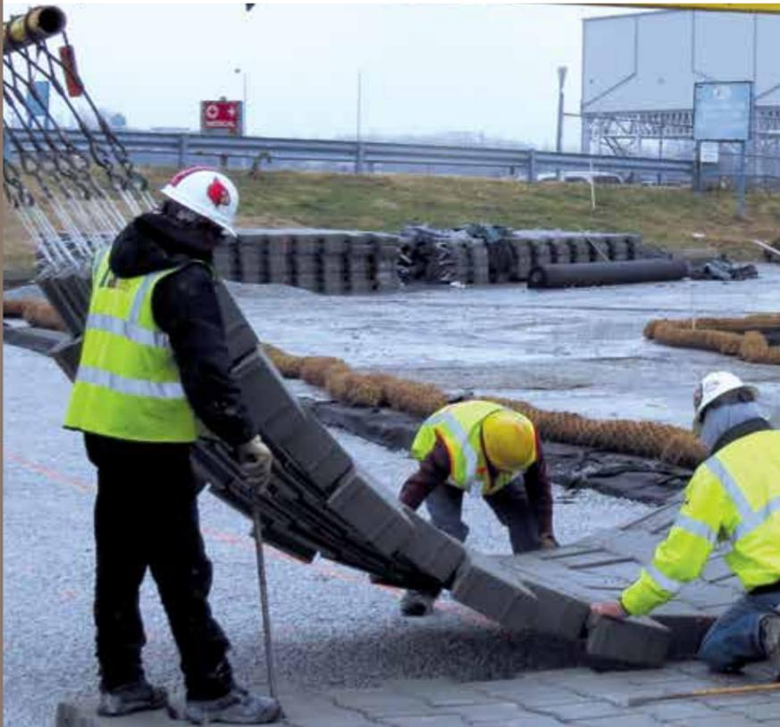
The *PaveDrain* System allows for more installation flexibility than ANY paving product available on the market today. Mat installation is done with conventional construction equipment (excavator, crane, forklift, etc.) and 3-4 laborers.
