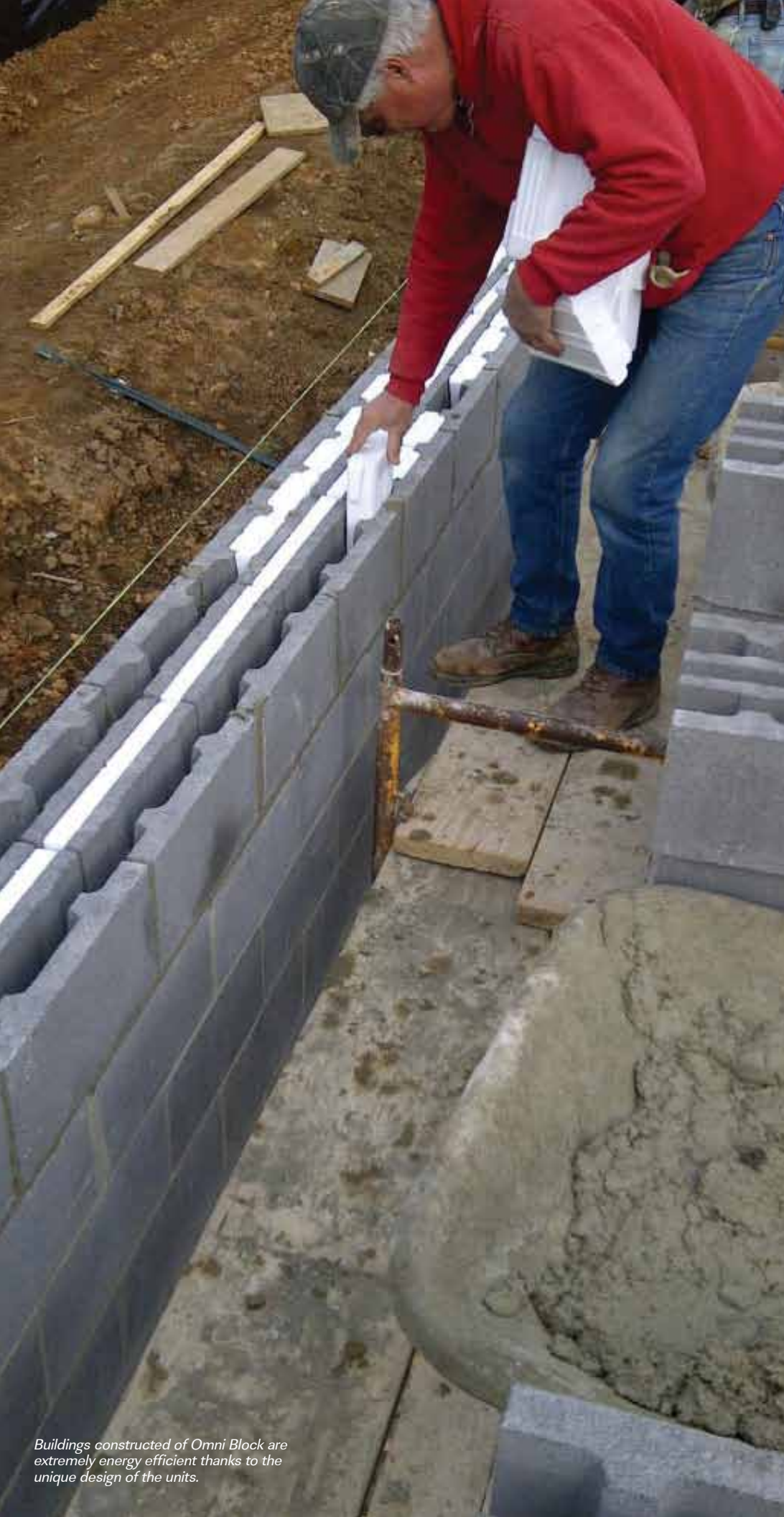
Several Omni Block sizes and configurations have been engineered to provide the optimum design for unit application. (12" Omni Block Unit shown)
