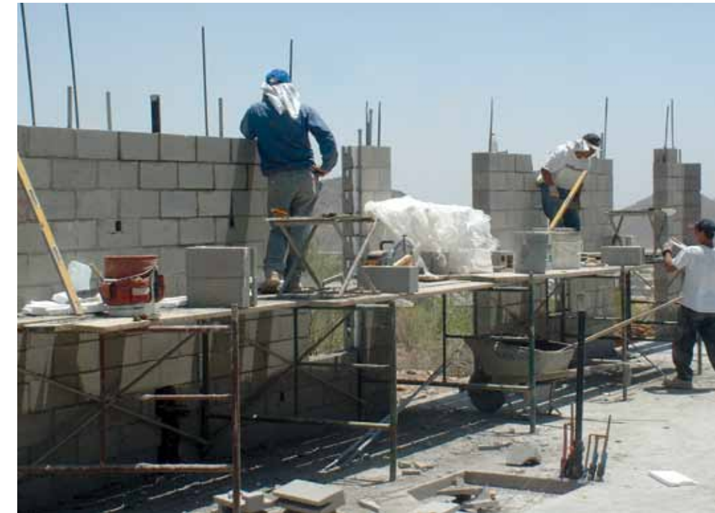
The Omni Block is a patented insulated concrete masonry unit (CMU) wall system which combines the benefits of indigenous aggregates, Expanded Polystyrene, thermal lag, exposed thermal mass and air tightness resulting in a highly thermally efficient wall system.
